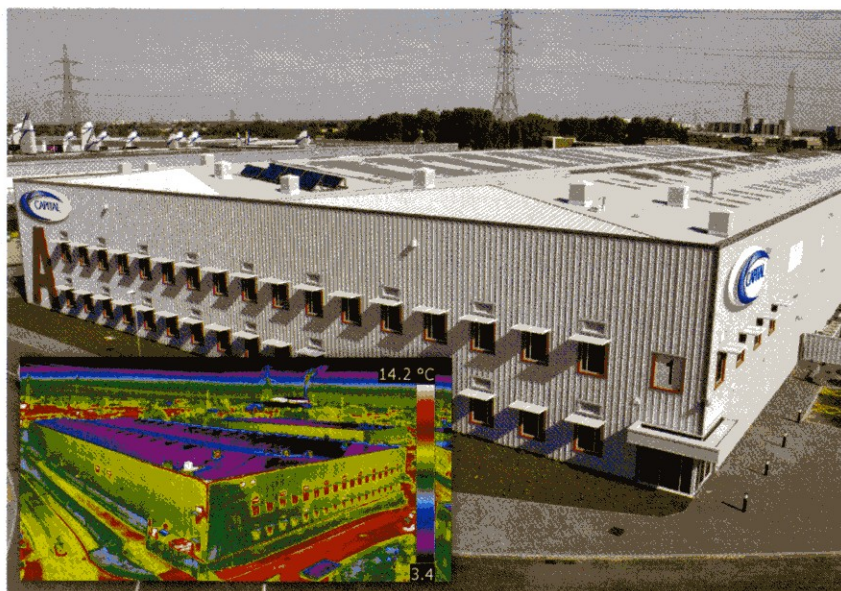
Capital's new Beckton Waterfront site was designed with energy saving and recycling features in mind; (inset) a thermal image of the Capital building demonstrating its energy efficiency
